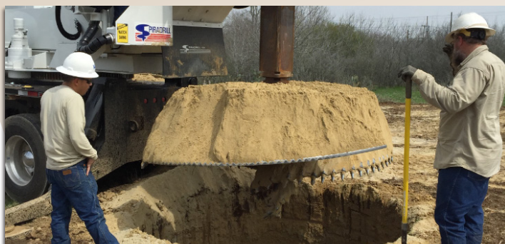
As part of the Capote to Deer Creek rebuild, crews drill the structure foundation for the new 138kV transmission line.
