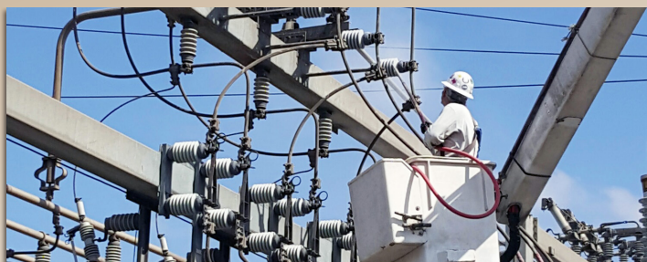
The CMC substation undergoes a biannual cleaning of its equipment. Maintaining the health and cleanliness of GVEC infrastructure extends equipment life and ensures reliability.
