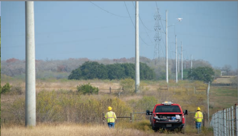
At GVEC, we continue traditional ways of ensuring optimal performance of our distribution circuits while also embracing new technology. Drones are helpful tools in inspecting and identifying trouble spots along our lines.
