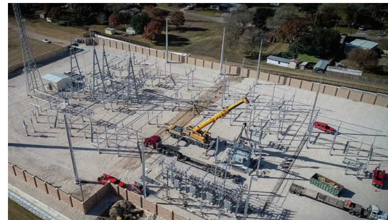
The Meadow Lake Substation, constructed with a 180-foot communications tower, is an example of technologies working together, supporting fiber-based communication and future FTTH buildouts. It’s the first GVEC substation with a separate communication and network room to give better accessibility and with backup power using a more efficient and robust DC power plant.
