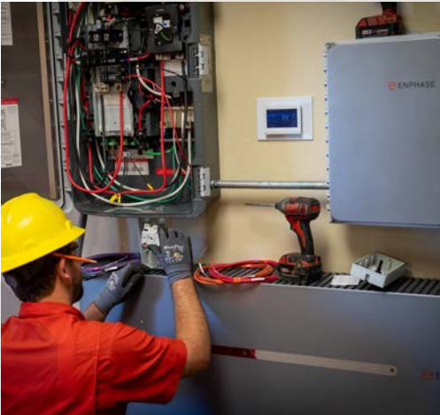
A member of GVEC's Electrician team works on the installation of a home solar panel and battery storage system.
